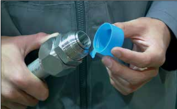
Bring the tube to installation site. Remove the plastic plug from the tube end.
