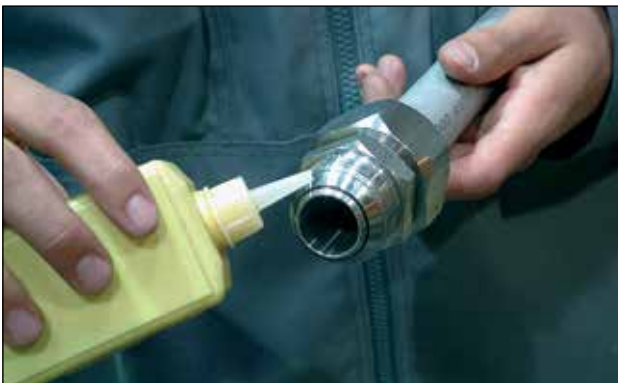
Use oil on the nut, body and the flared tube end. For stainless steel use Molybdenum Disulphide or other antiseize lubrication. Lubricate O-ring with oil.
