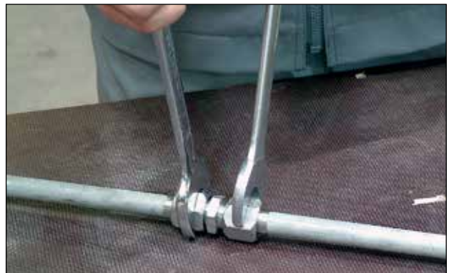
After hand tightening use a spanner to tighten up 1/4" to 3/4" turn. Make up the nut fully. Do not wait till later to tighten up. The tube shall not rotate during tightening.
