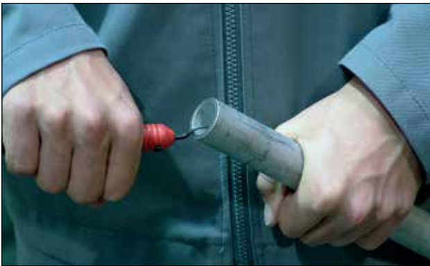
The pipe is first deburred inside and out.
