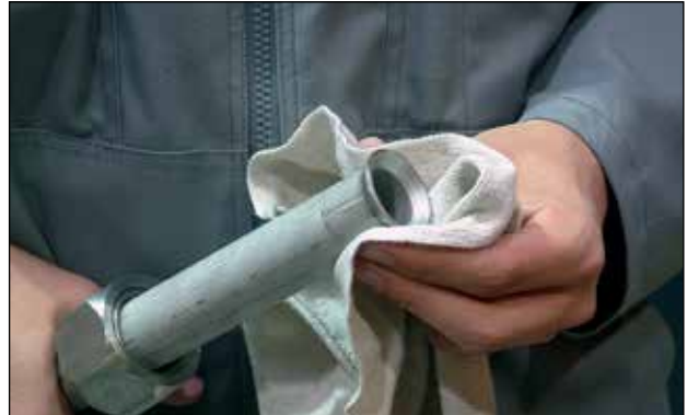
Clean the flared tube with clean cloth.
